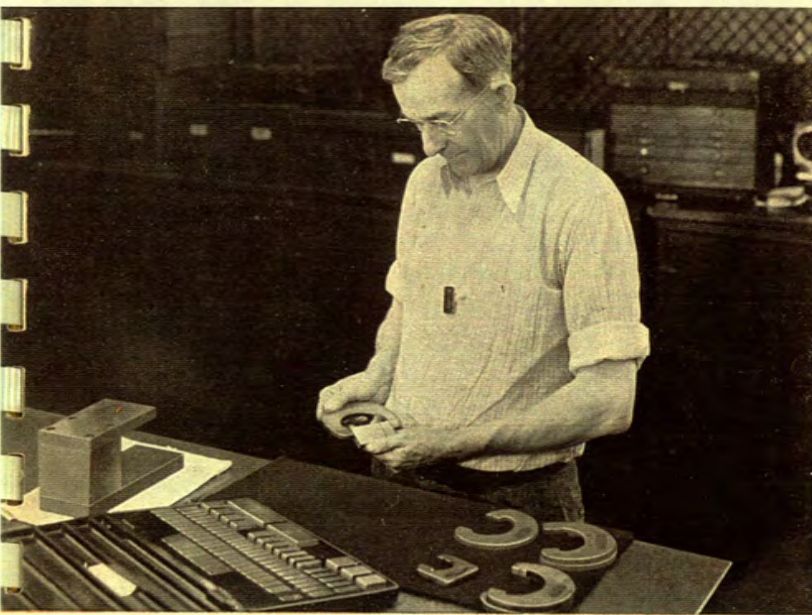
Precision manufacture. Johansson gages, magical blocks of steel, accurate to within two-millionths of an inch, test all shop and working gages in the Lincoln-Zephyr plant.
